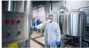
Production Industrial refrigeration
